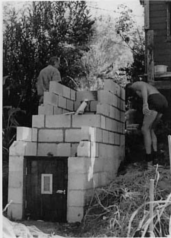
FIG. 18 Stepped footing option
