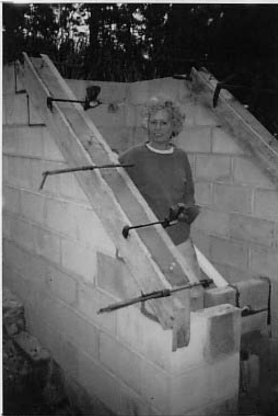
FIG. 19 Finishing sloping walls
