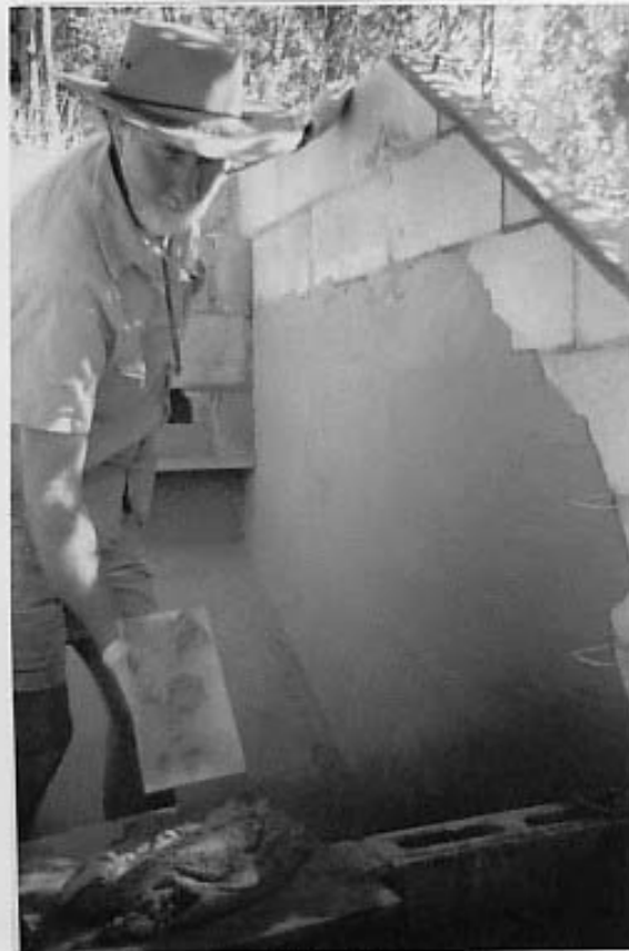
FIG. 20 Rendering inside of chamber
