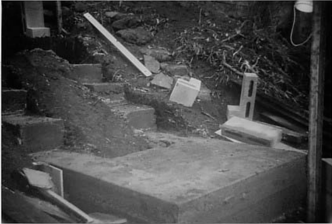
FIG.11 Stepped footing & humus chamber floor
