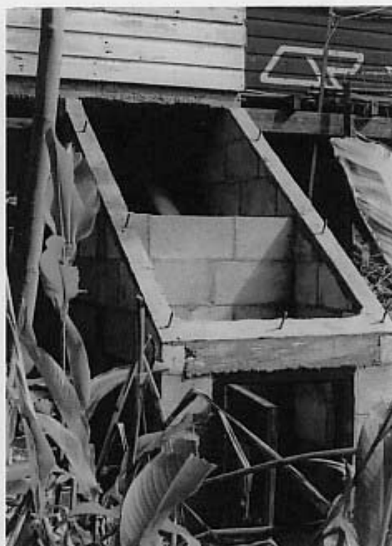
FIG. 16 Top ready for fixing iron
