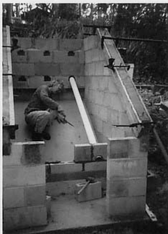
FIG. 15 Vent pipes, finishing sloping top (wide chamber)
