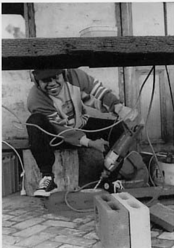
FIG. 13 Drilling holes in blocks
