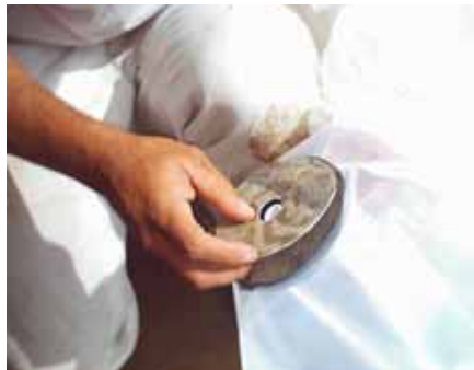
Above: Installing the washer assembly in the digester bag.
