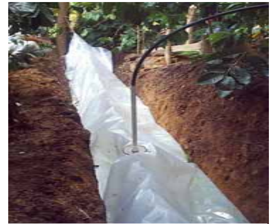
Above: Bio-digester bag is hanging between two trees while filling with water.
