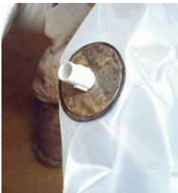
Above: Installing the washer assembly in the digester bag.
