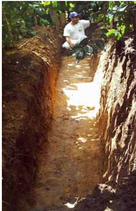
Above: Bio-digester trench
